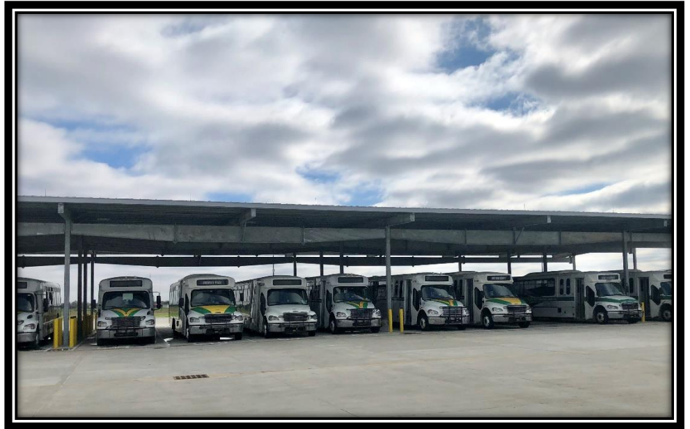
Covered Parking for Bus Fleet
