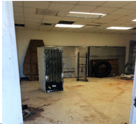
Photo 3 General view of back storage room.
