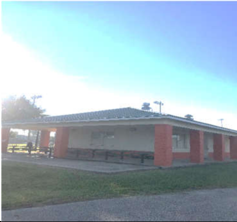
Photo 1 View of building exterior.
