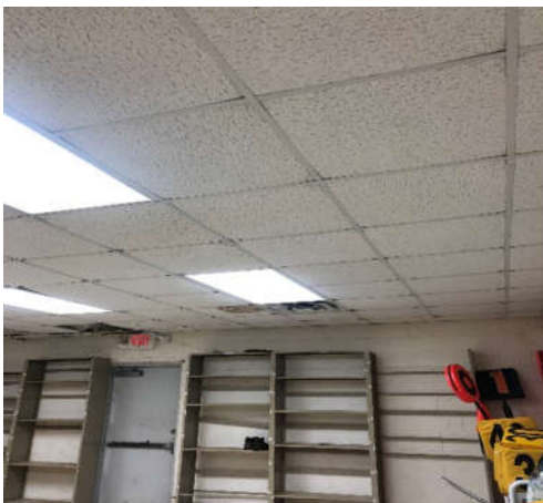
Photo 5 View of 2'x2' ceiling tiles.
