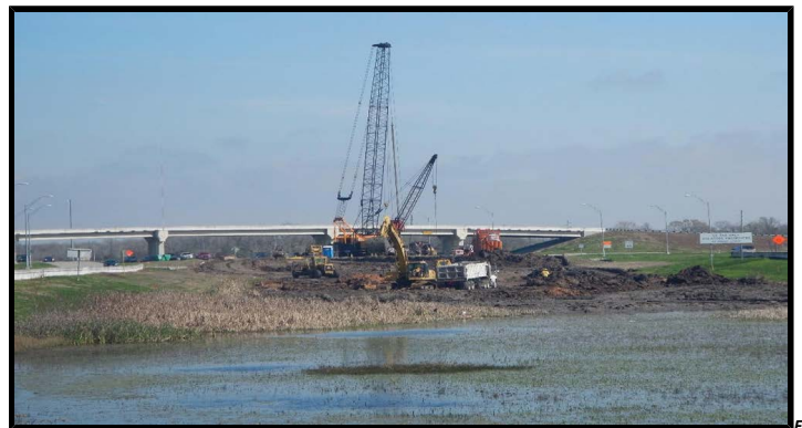
Bend Parkway Highway 6 Overpass – drill shaft foundation installation
