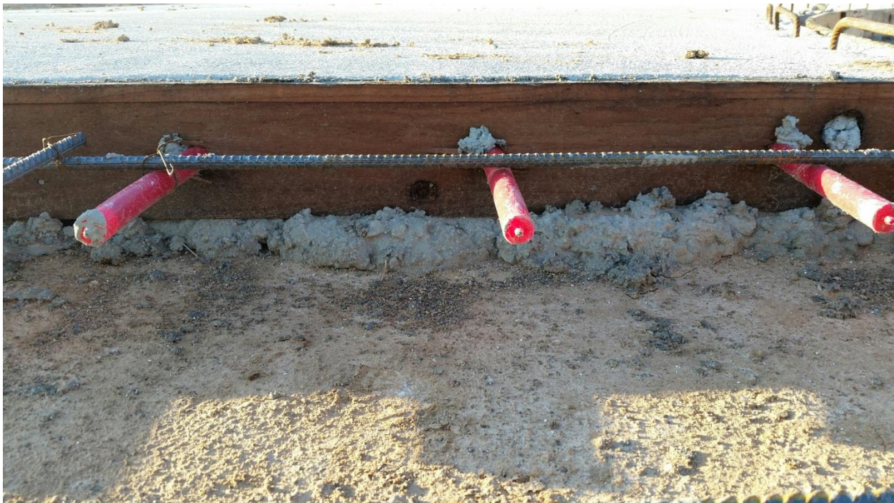
Image 8 - Concrete under headers at expansion joints does not allow expansion to occur correctly.
