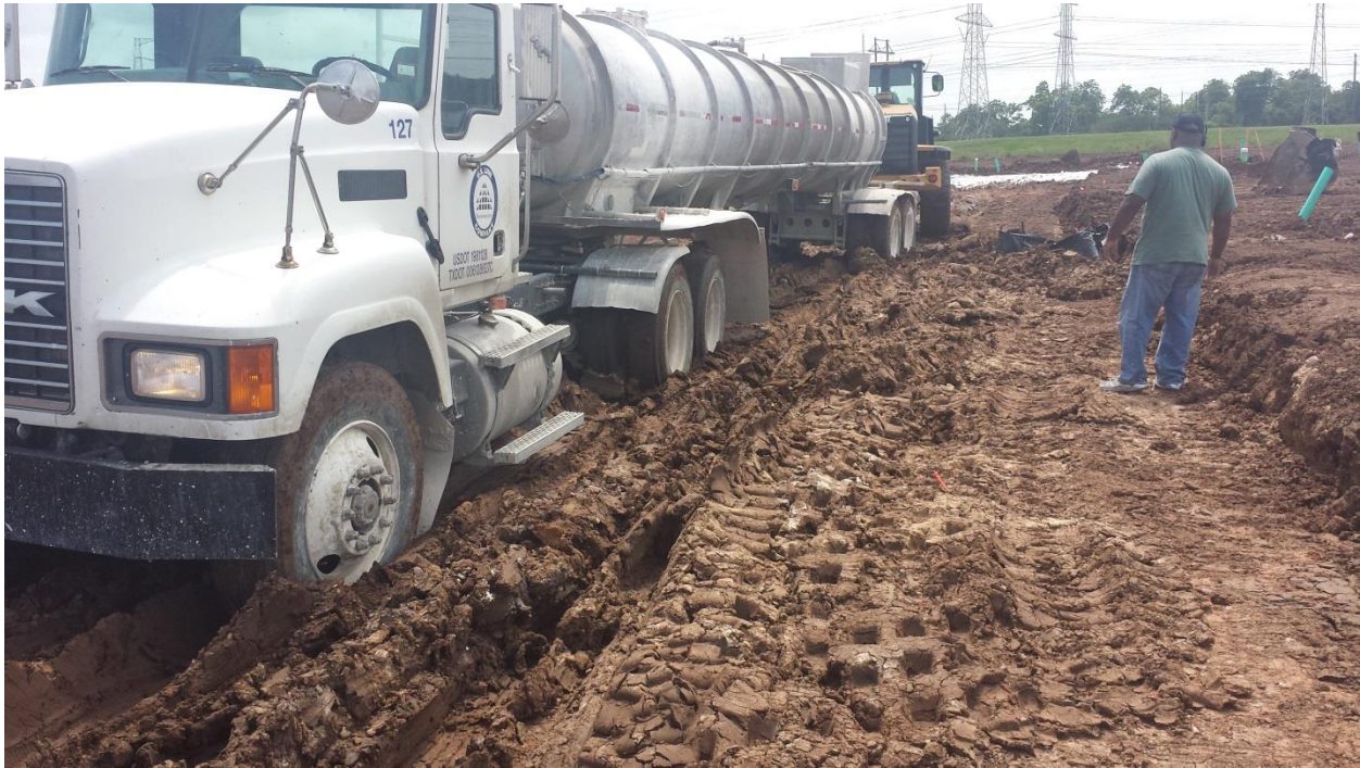
Image 7 - Possible deficiencies in subgrade and base include: Inadequate proof rolling or improper mixing of lime for subgrade, not extending lime mixture to edges of proposed limits of the stabilized subgrade, calculating lime for a 6 inch subgrade and mixing it 8 or more inches deep.
