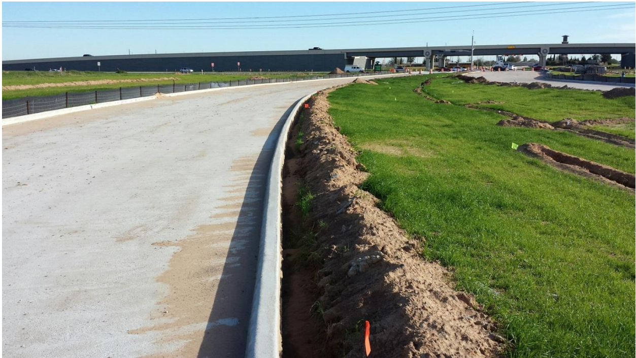
Image 13 - Silt fence or irrigation is placed directly behind curb cuts through subgrade and impacts lateral support.
