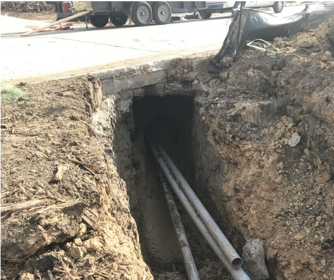
Image 18 – Private utility excavation beneath pavement
