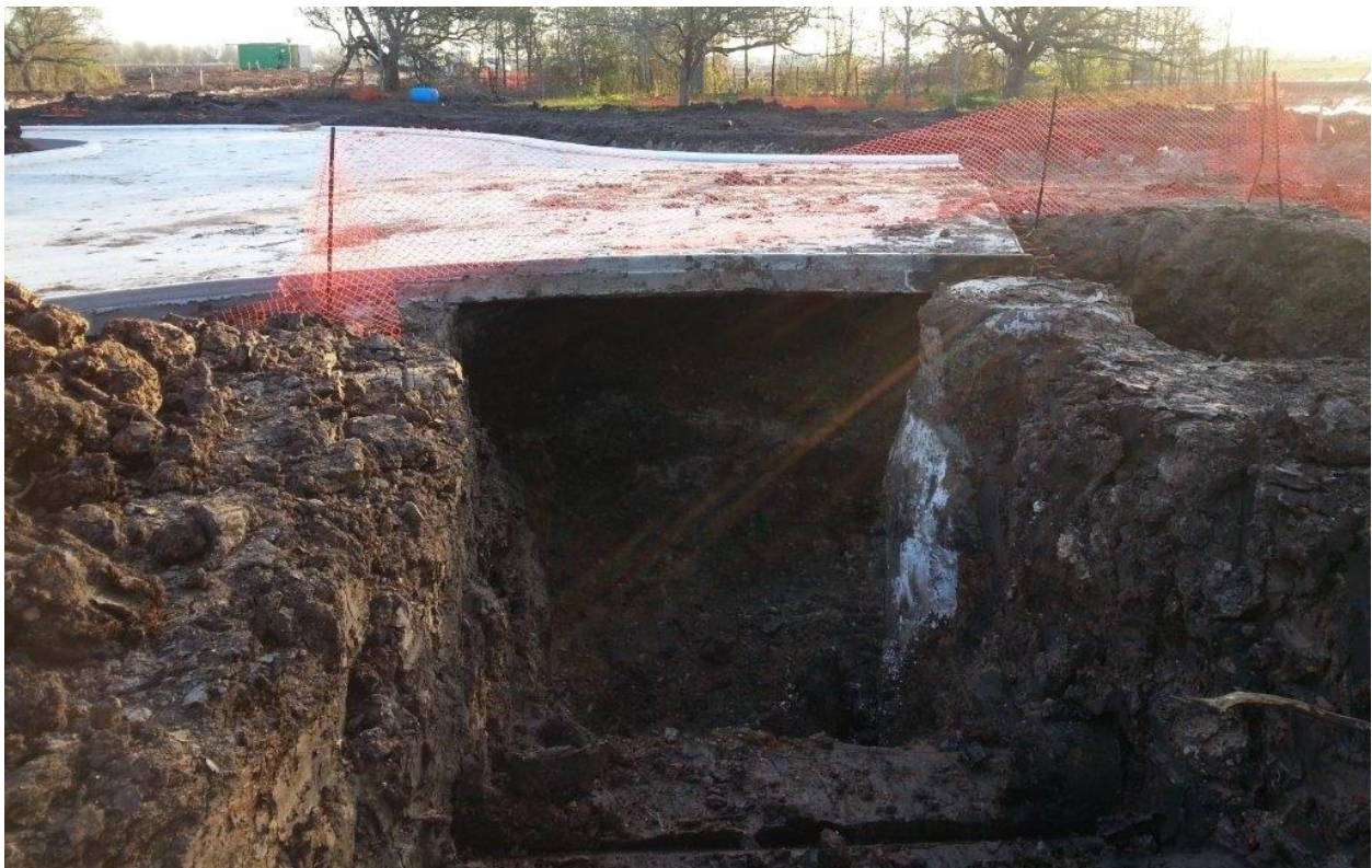
Image 14 - Excavation under or near pavement
