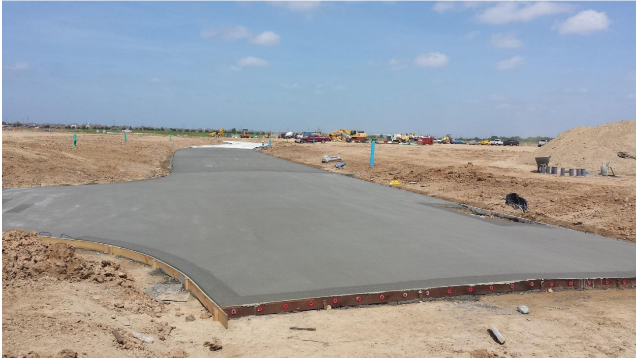
Image 11 - Membrane curing compound not applied to pavement
