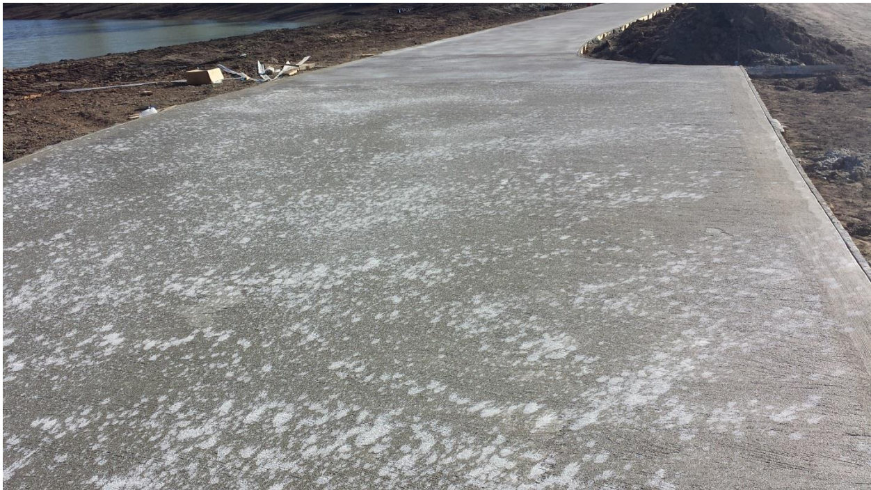
Image 12 - Inadequate curing compound
