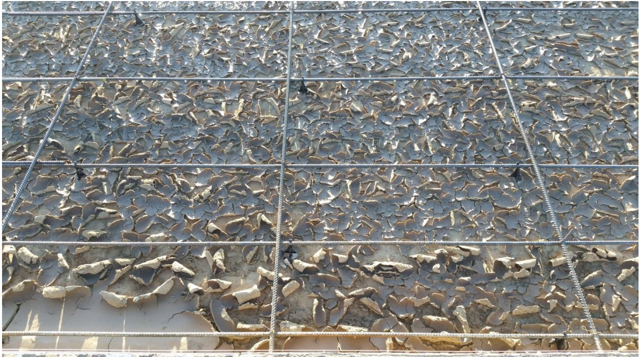
Image 6 - Subgrade is too dry.
