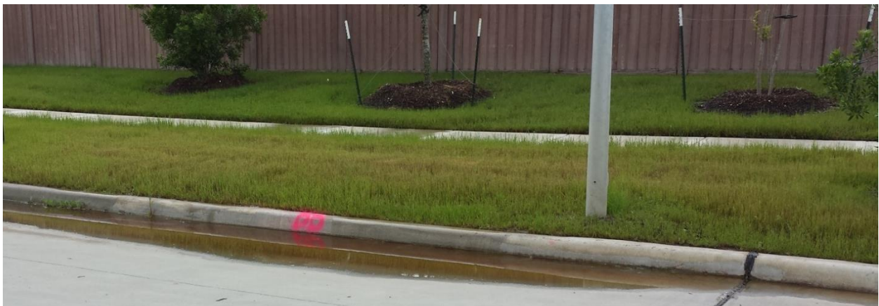
Image 2 - Bird bath has significant length and depth. Lifting, light grinding, or removal of joint sealant obstruction may be acceptable based on field conditions. Grinding shall be limited to 15' either side of the expansion joint.
