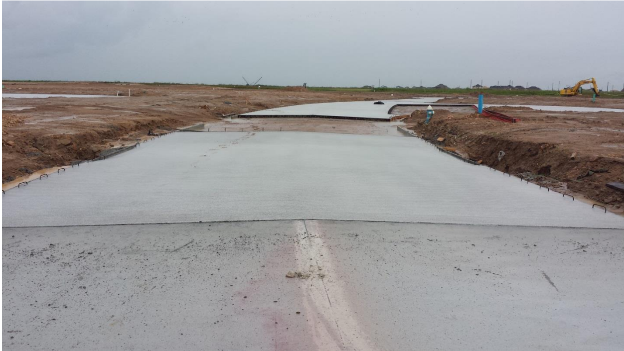
Image 15 - Not saw cutting within specified time (photo shows 4 day old concrete with no sawcuts)
