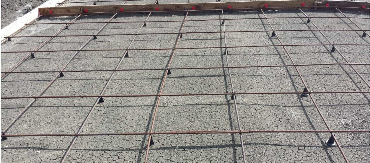
Image 5 - Subgrade is too dry.
