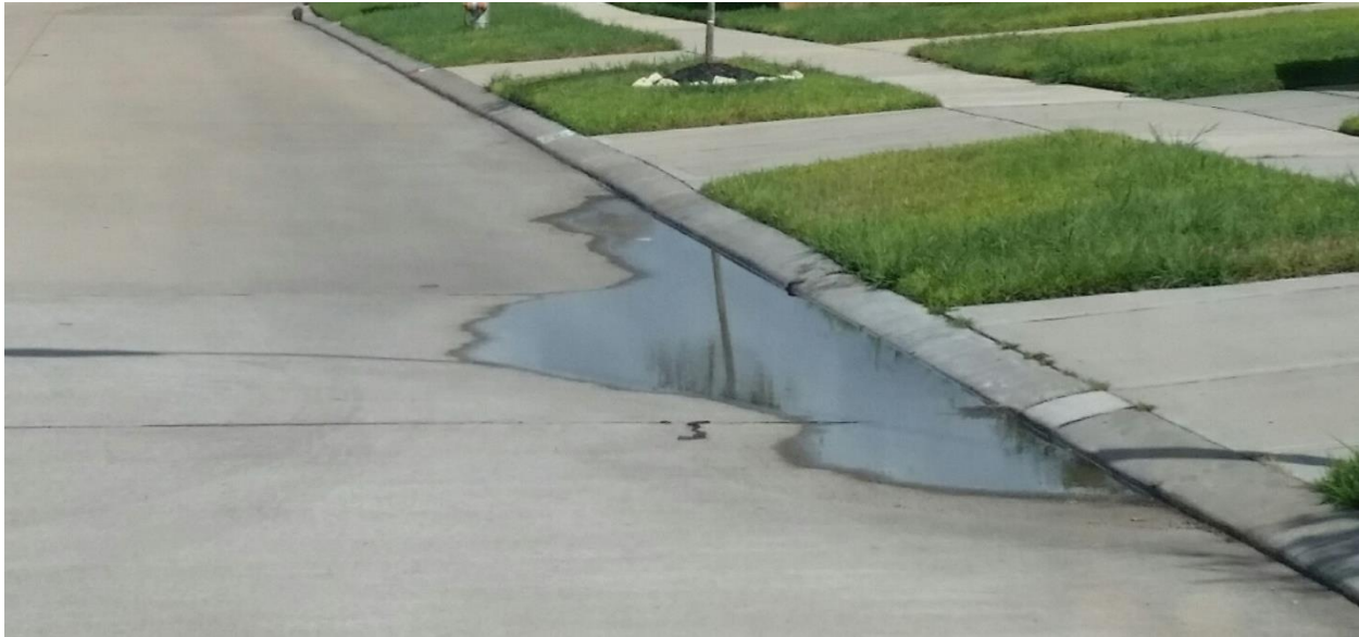
Image 3 - Bird bath has significant length, width, and depth. Lifting or pavement replacement is required. If the lifted pavement cracks then use Concrete Pavement Cracking Evaluation Criteria included in this document.
