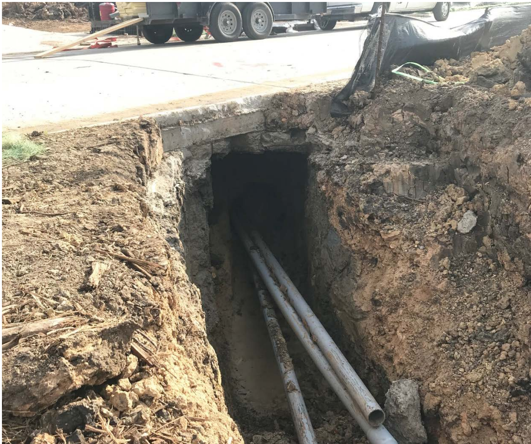
Image 18 – Private utility excavation beneath pavement
