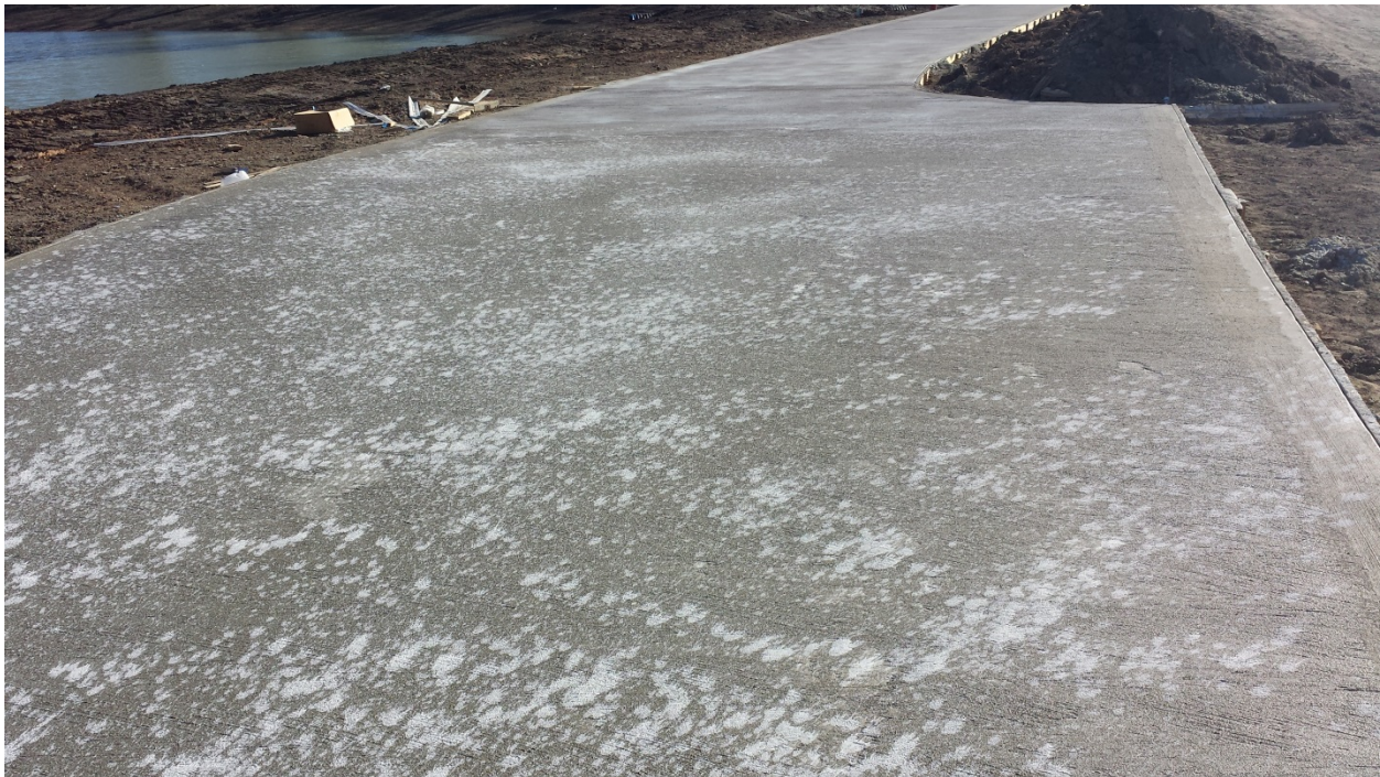
Image 12 - Inadequate curing compound
