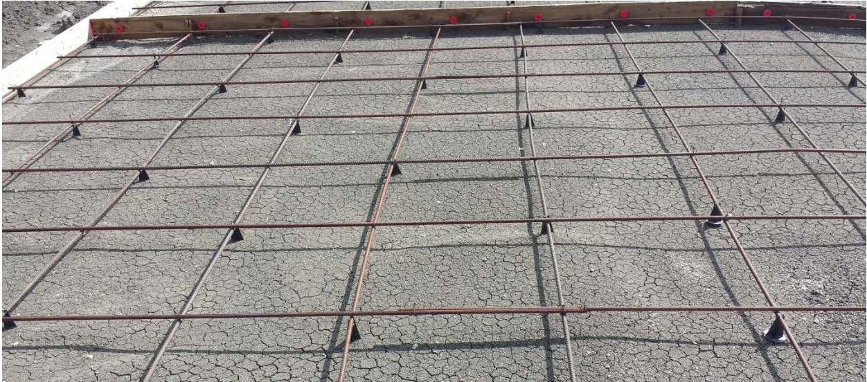
Image 5 - Subgrade is too dry.
