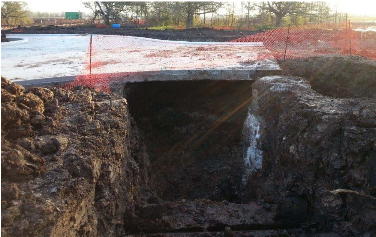
Image 14 - Excavation under or near pavement
