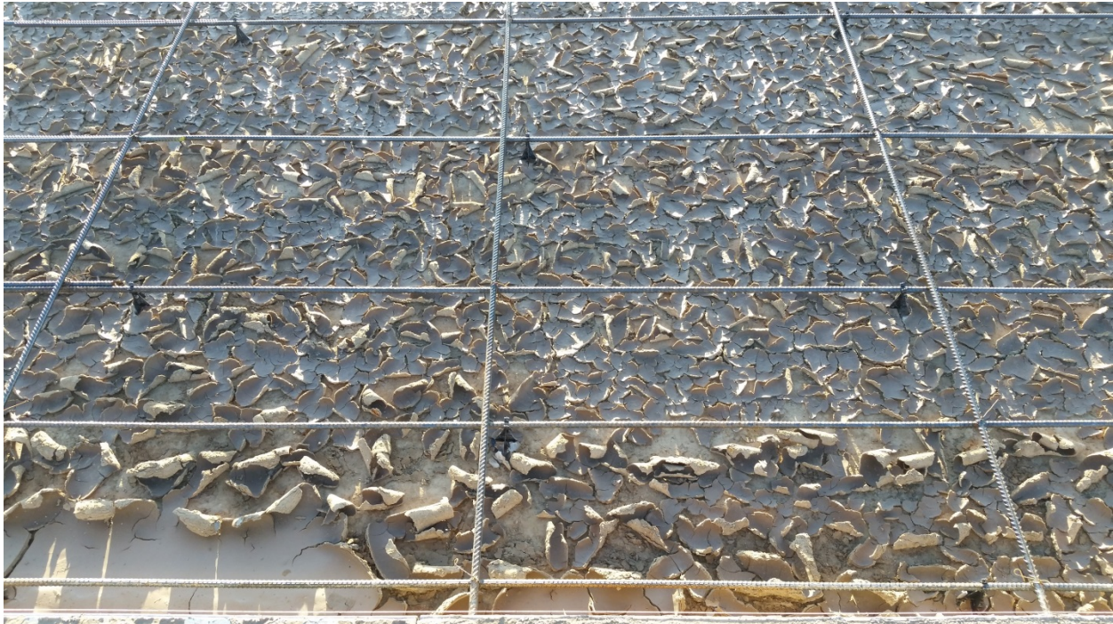
Image 6 - Subgrade is too dry.
