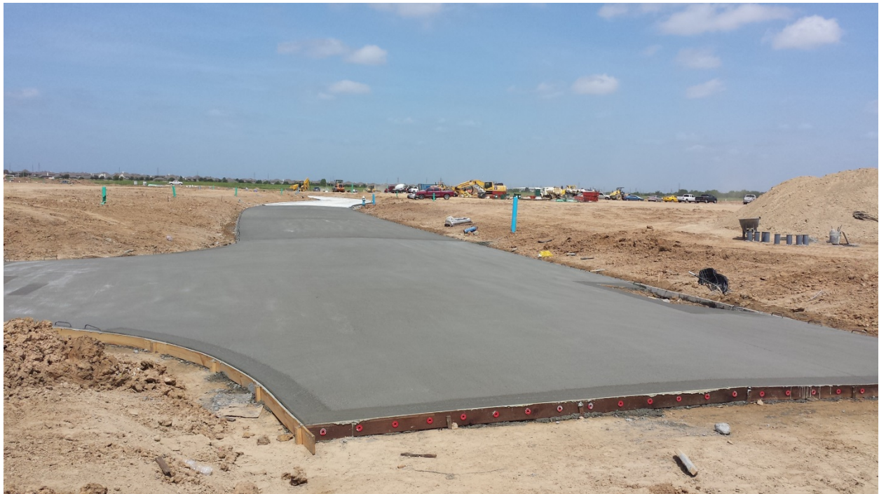
Image 11 - Membrane curing compound not applied to pavement
