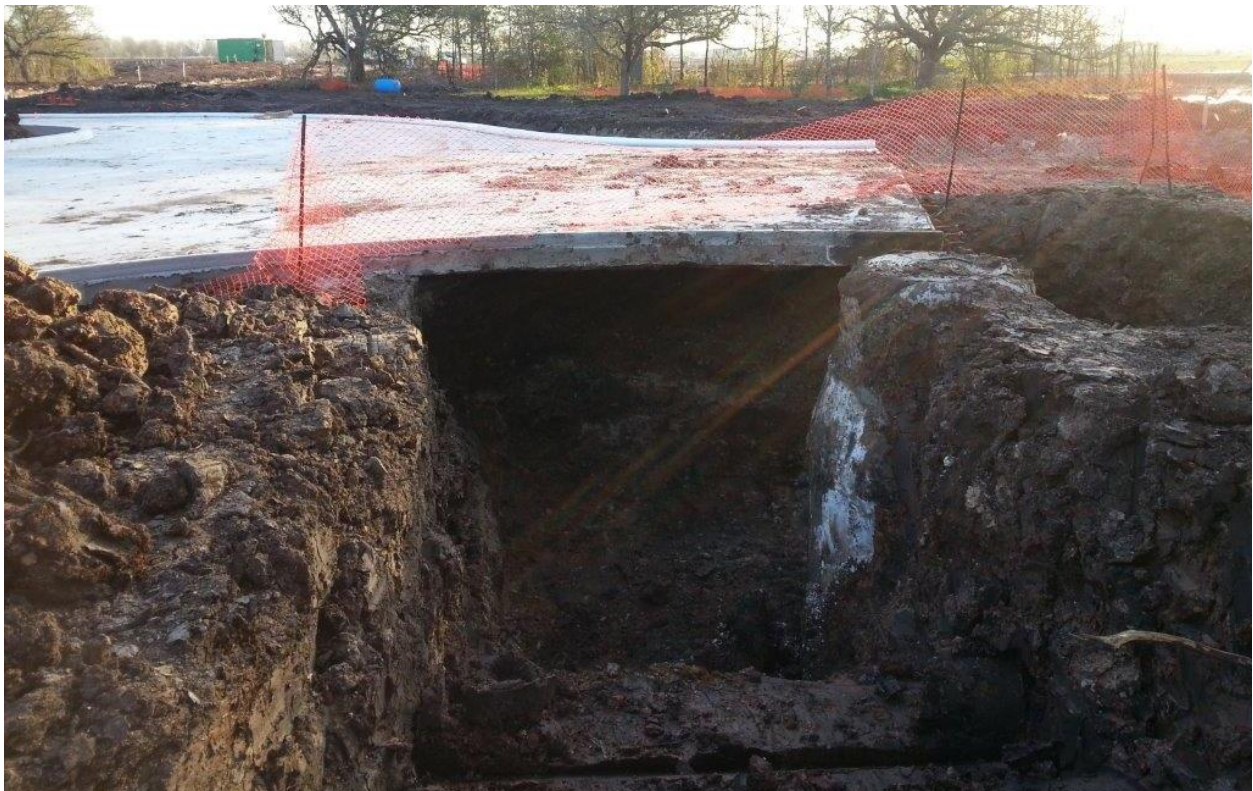
Image 14 - Excavation under or near pavement
