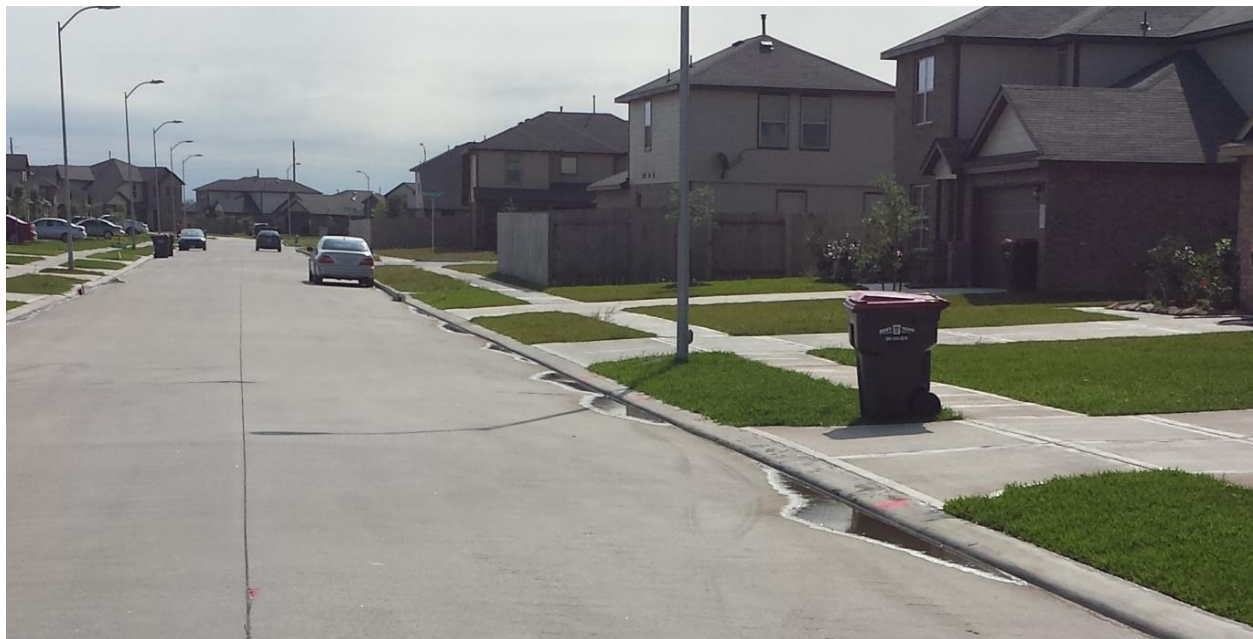
Image 4 - Bird baths which are relatively small in length, width, and depth do not require pavement replacement or lifting. Allowable width is approximately 12 inches.
