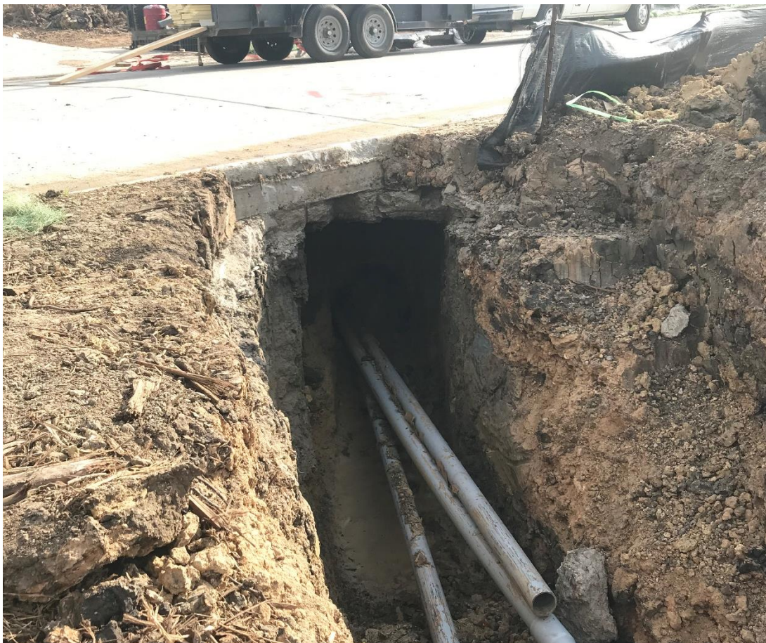
Image 18 – Private utility excavation beneath pavement
