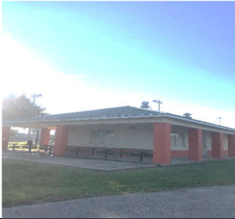
Photo 1 View of building exterior.
