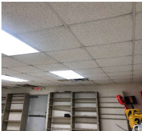
Photo 5 View of 2'x2' ceiling tiles.
