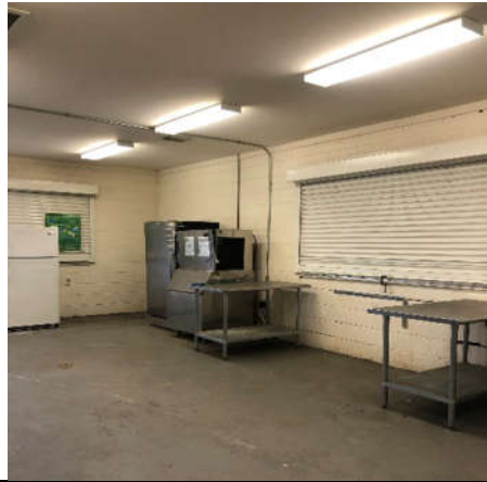
Photo 2 General view of kitchen.
