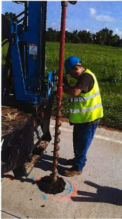
Pic. 1: Drilling at B-4
