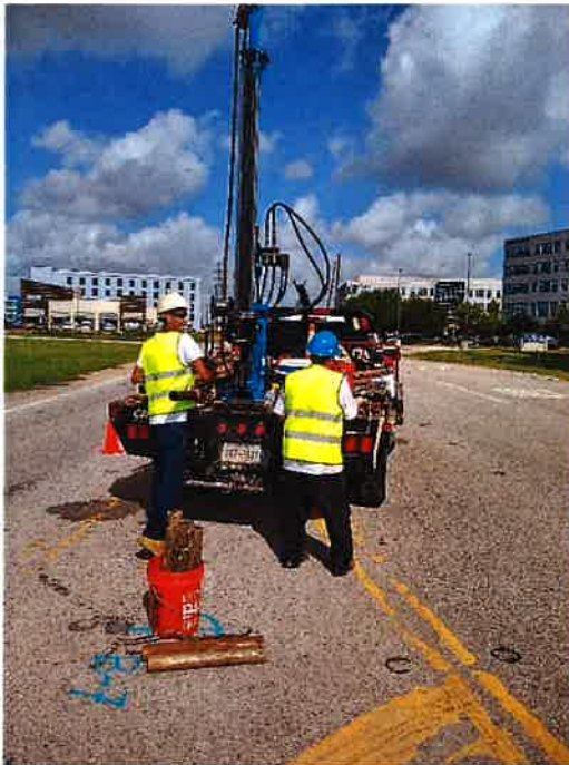
Pic. 3: Drilling at B-7
