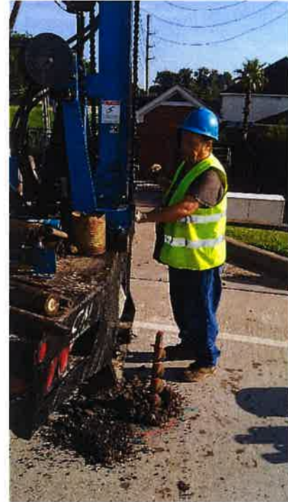
Pic. 2: Drilling at B-5
