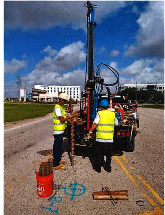
Pic. 4: Drilling at B-7
