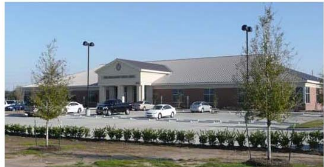
Precinct Three Annex
