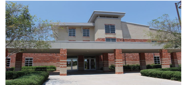
Training Facility—Sienna Annex
